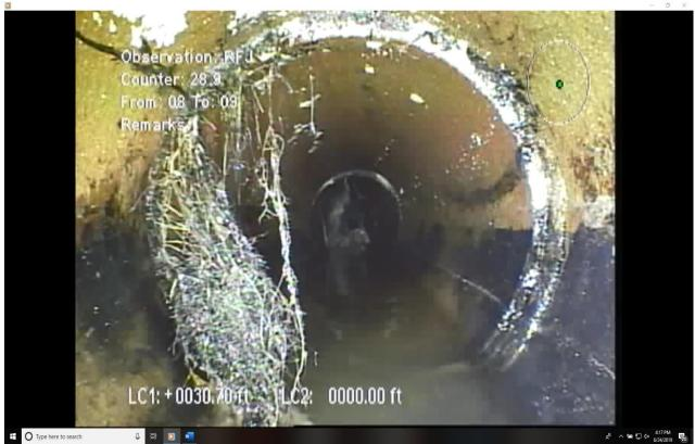
As previously stated, the City encountered an obstruction at approximate STA 0+34 during their jetting operations on June 20<sup>th</sup>. As shown below in Photo #4, large amounts of roots and debris were still present at STA 0+34 following the jetting operation.
