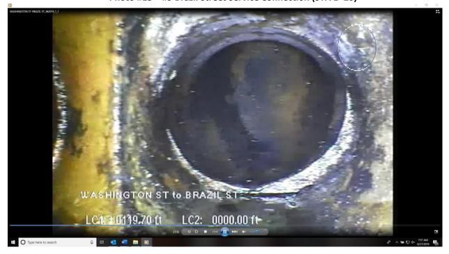
Grease or Indications of grease and surcharging (black staining) were also present in the service connections from #12, #13, and #18 as shown in the following photographs as observed from the 6-inch sewer main.
