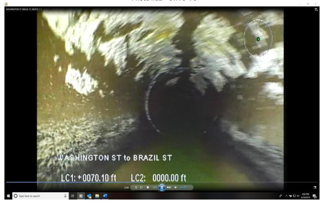
In addition to the grease and debris present in the previous photos, "black staining" can be seen along the sides and near the top of the pipe. Such staining is indicative of wastewater flows being at this level for long periods of time. It appears to be a systemic problem in the existing Brazil Street sewer and not one that recently developed.
