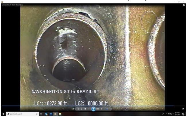
In addition to the roots, grease and pipe surcharging, numerous structural issues were found during the CCTV inspection of the existing Brazil Street sewer. A total of 19 locations were identified with one or more of the following structural issues:
