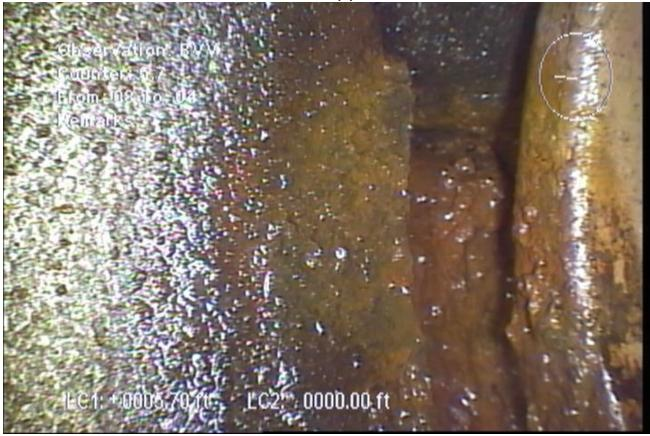
Photo #23 – Spiral crack at STA 1+31
