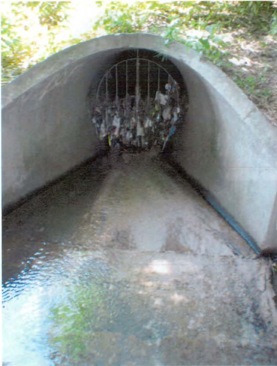
Note off-white filamentous bacterial growth
