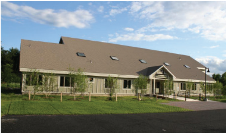
Figure 2: New England Environmental, Inc. with porous asphalt drive in foreground and grass paver parking stalls in middle ground | Courtesy: Mickey Marcus, NEE
