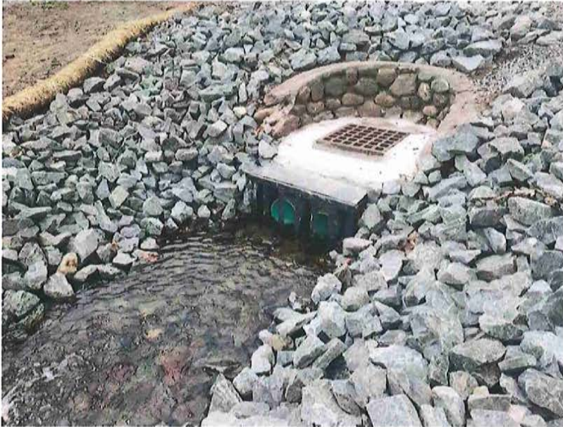
Inlet on Towners Pond side
