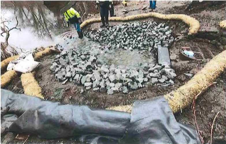
Swains Pond Ave. – Culvert replacement
