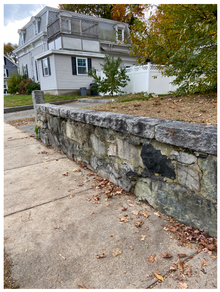
EXISTING STONE WALL AT FRONT OF PROPERTY TO REMAIN
