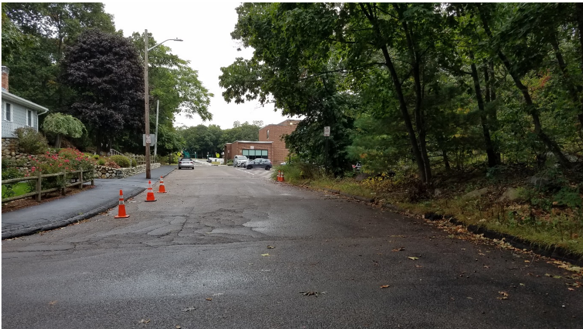
Hawthorne Road - Hoover School Property (facing north)
