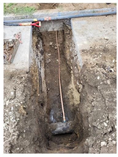
of the replacement. The DPW will also confirm the material on the public side (from the property line to the main). The public-side services identified as lead will be excavated and replaced with copper by the DPW. Residents will receive 48-hour advance notice of planned water service shut down. This is a multi-year program, funded in part by the MWRA and the CWT.
