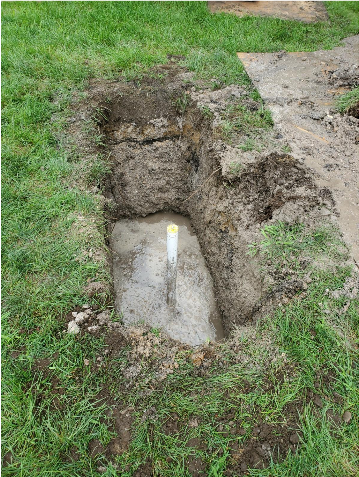
Photograph 1: TP-1 and Monitoring Well Installation
