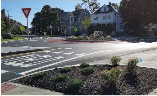
Figure 16: Roundabout at Green St. and Howard St. Intersection
