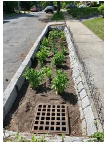
Figure 9: Rain Garden on Orient Ave.
