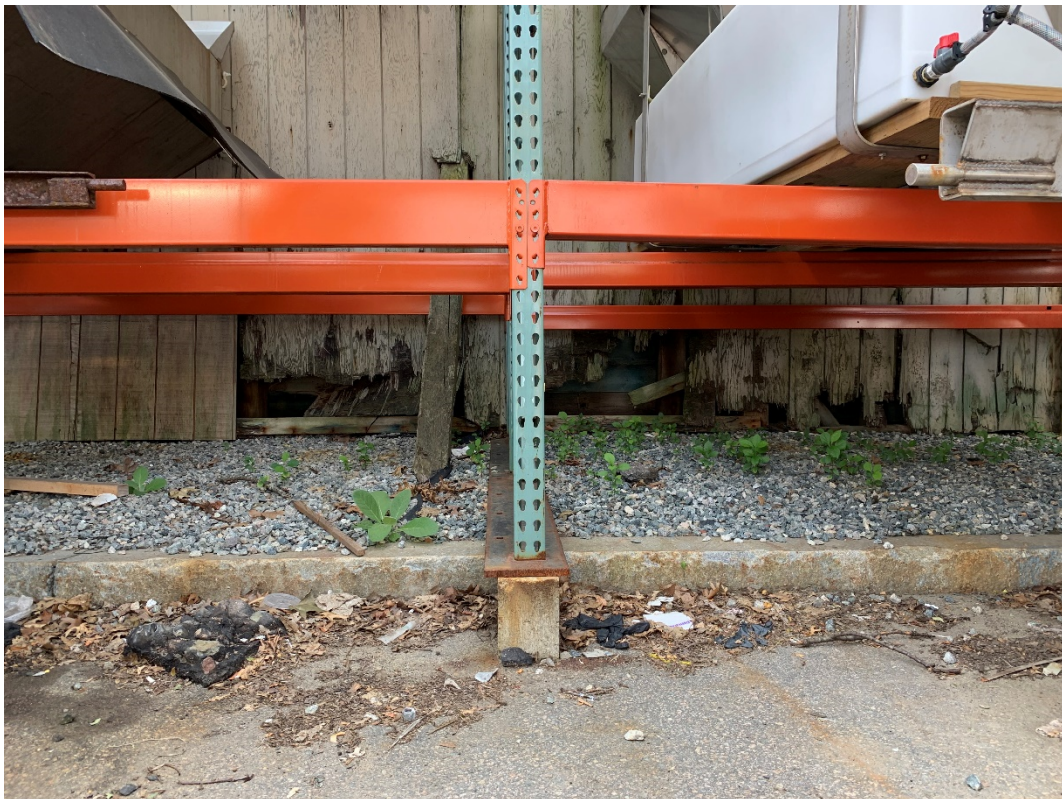
Photo 4: Typical deteriorated/damaged exterior wall panel
