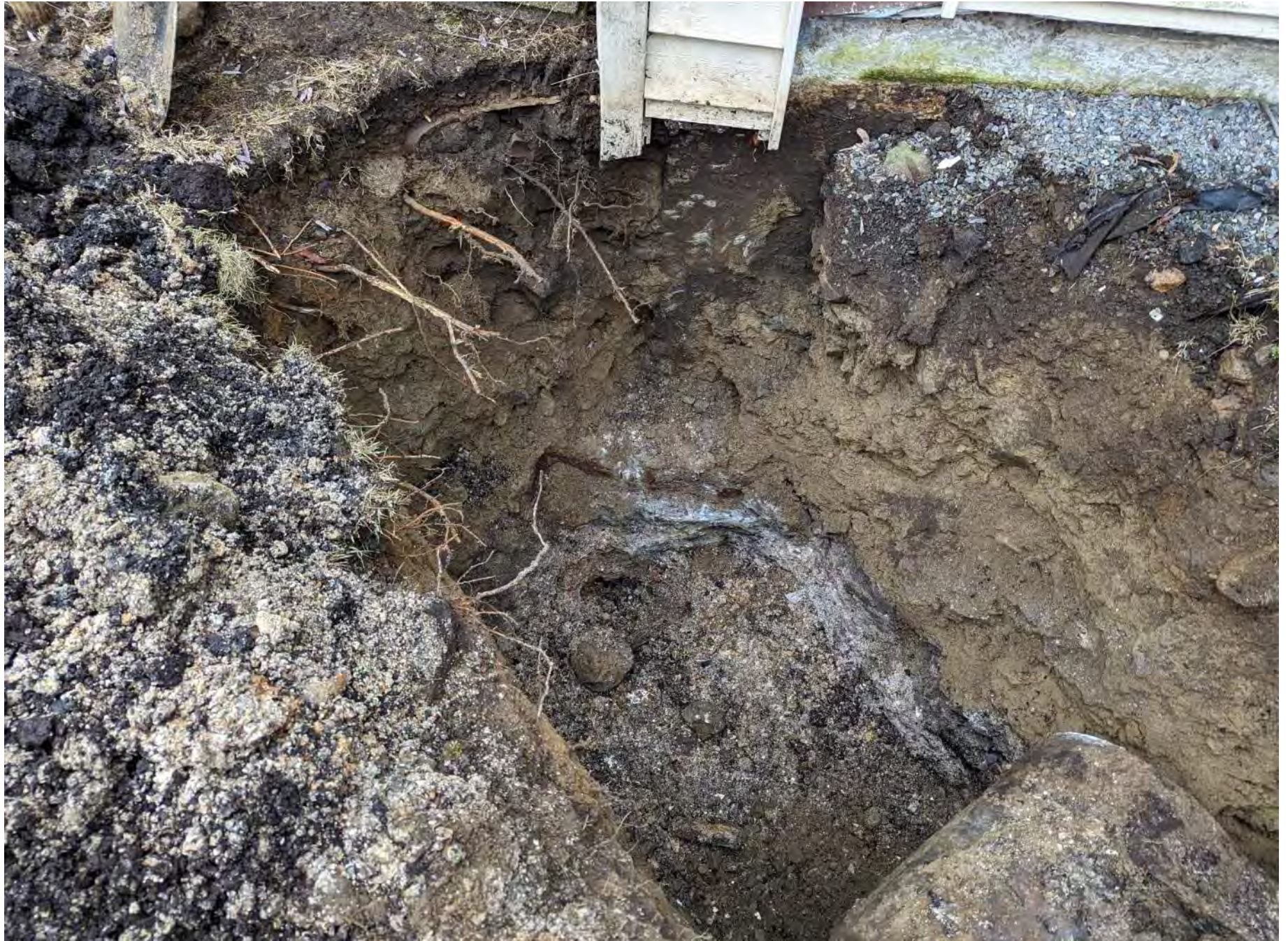
TP-1 VIEW LOOKING EAST
