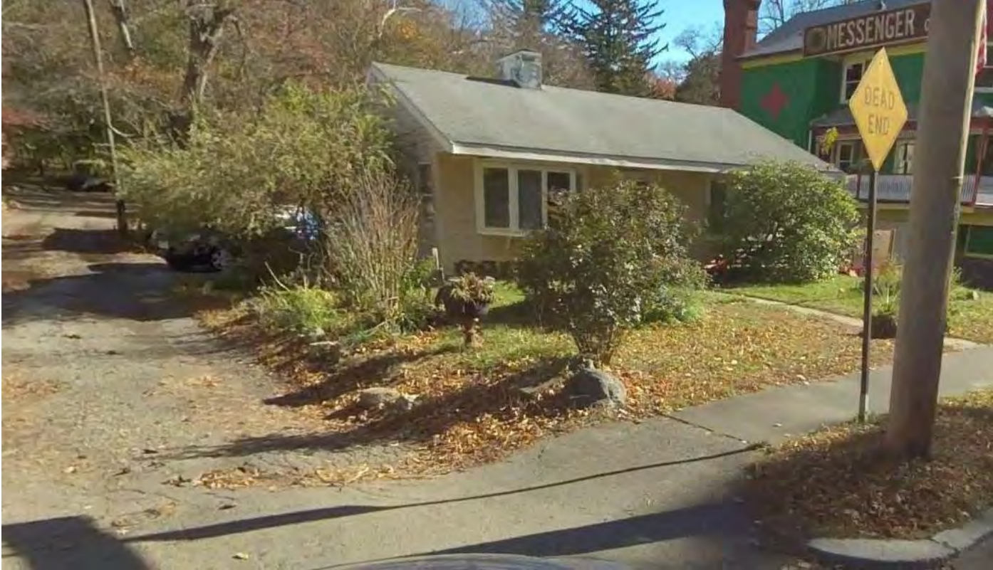
View of Site from Greenwood Street The existing structure is to be removed and replaced with a new dwelling .
