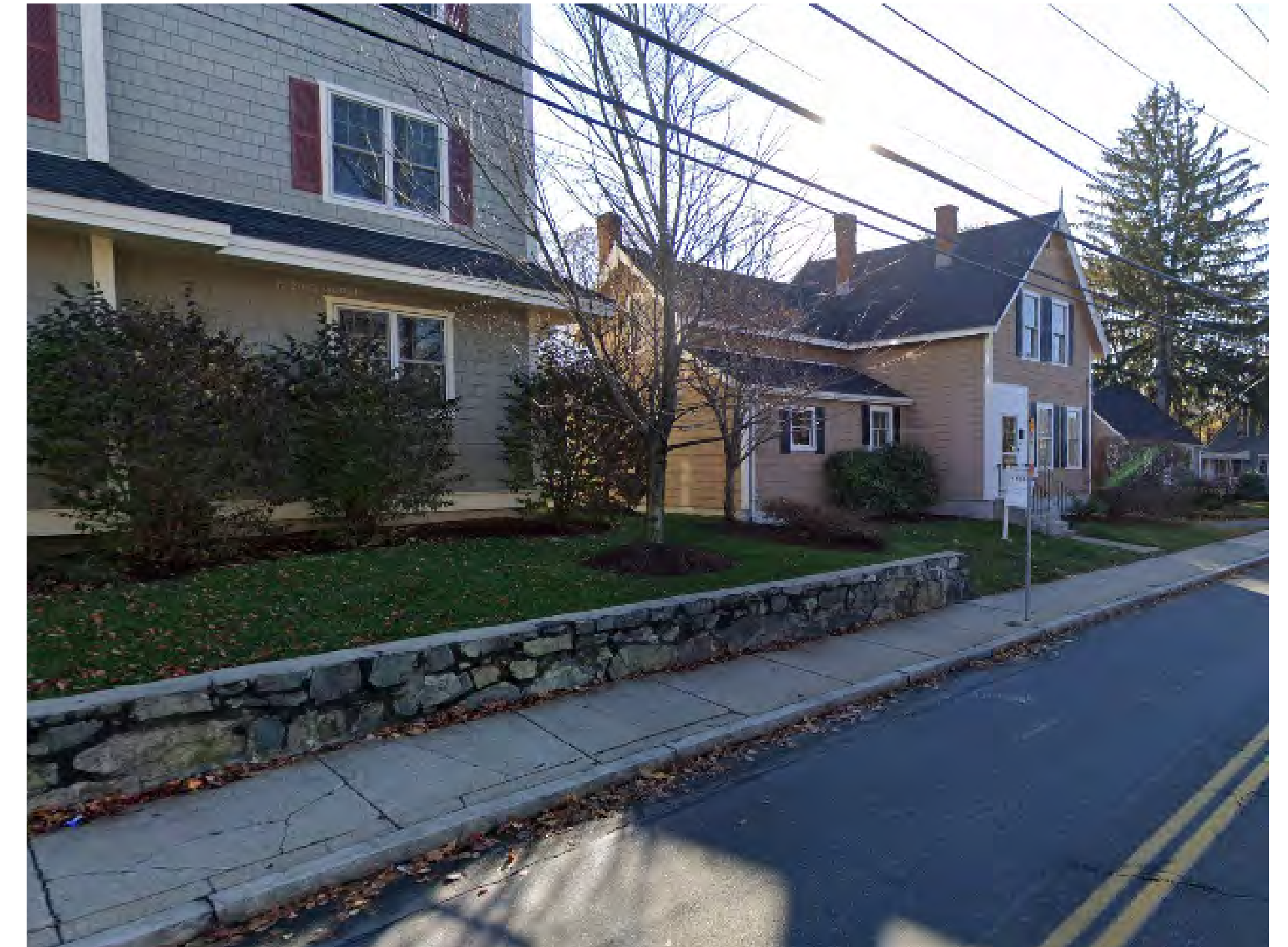
VIEW LOOKING WEST AT 373 PLEASANT STREET
