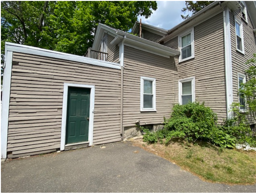
Appendix - existing condition photos
