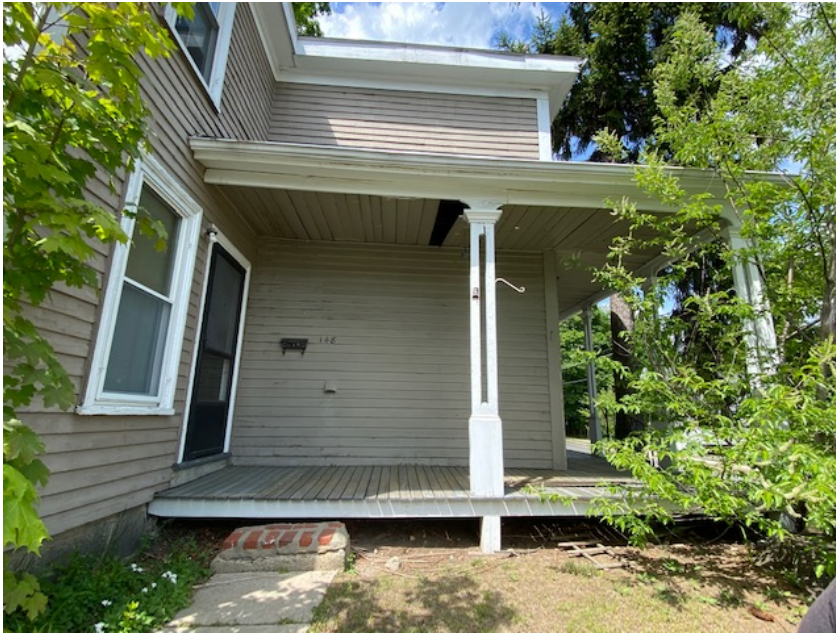
Exterior porch conditions
